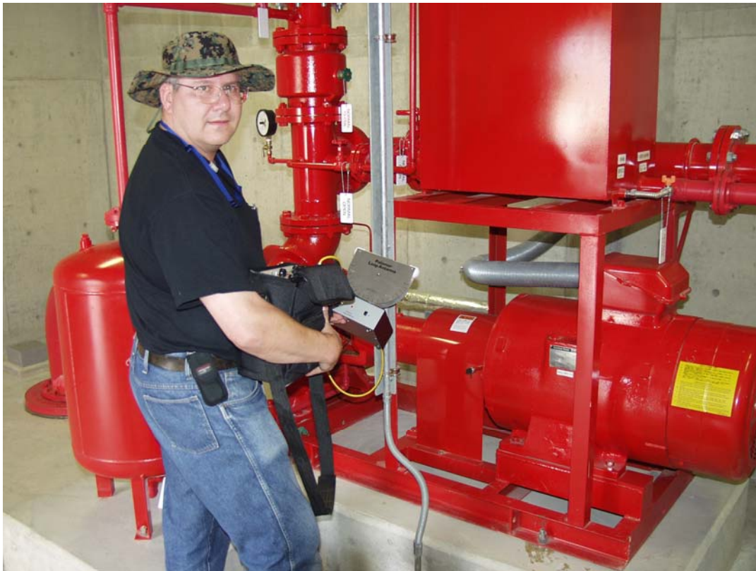
Figure 65 Using the Model 242 RFI Locator and Probe
