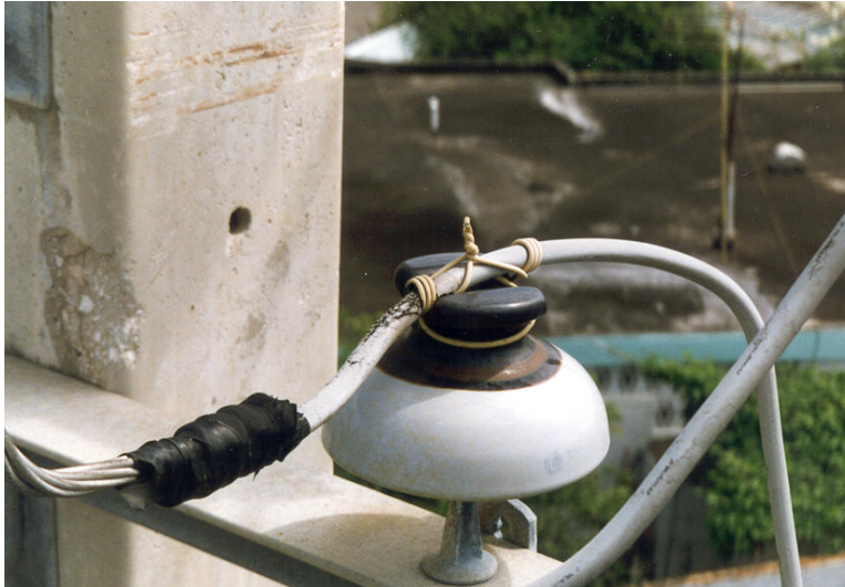
Figure 35 Insulated Tie Wire on an Insulated Conductor
