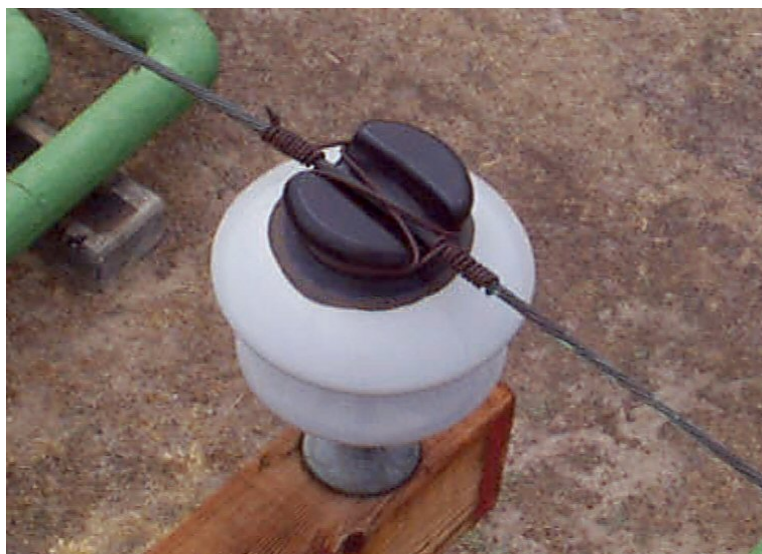
Figure 36 Insulated Tie Wire on a Bare Conductor
