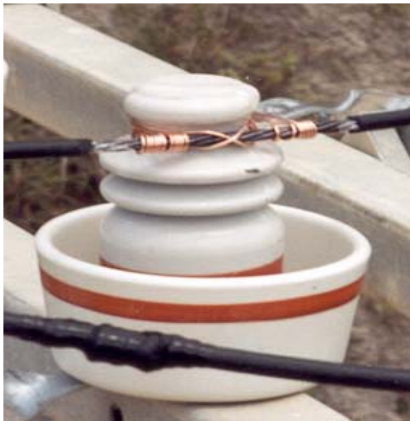
Figure 69 Tie Wire Source Mitigation, Example 2
