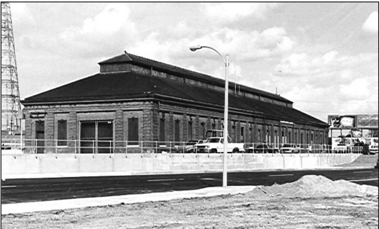
Figure 31. Drainage Pumping Station No. 1. View looking northwest.
