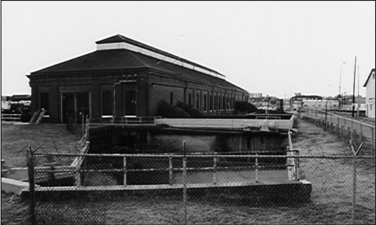
Figure 32. Drainage Pumping Station No. 1. View looking south.
