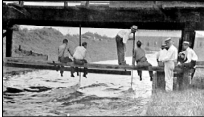
Figure 28. Testing of the 12' Wood screw pumps at Drainage Pumping Station No 1 (background), ca. 1915. Pitot tubes have been placed in the Metairie Relief Canal to measure the velocity of flow. This data was used to calculate the efficiency of the pumps. Tulane engineering students are holding the tubes while engineers record data (from Sewerage and Water Board 1915).
