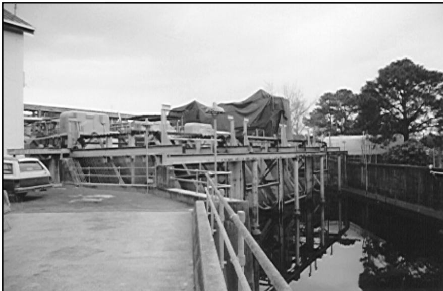
Figure 48. Drainage Pumping Station No. 4, viewed from the southeast. Pumping equipment is obscured by a tarpaulin; sandblasting in progress.
