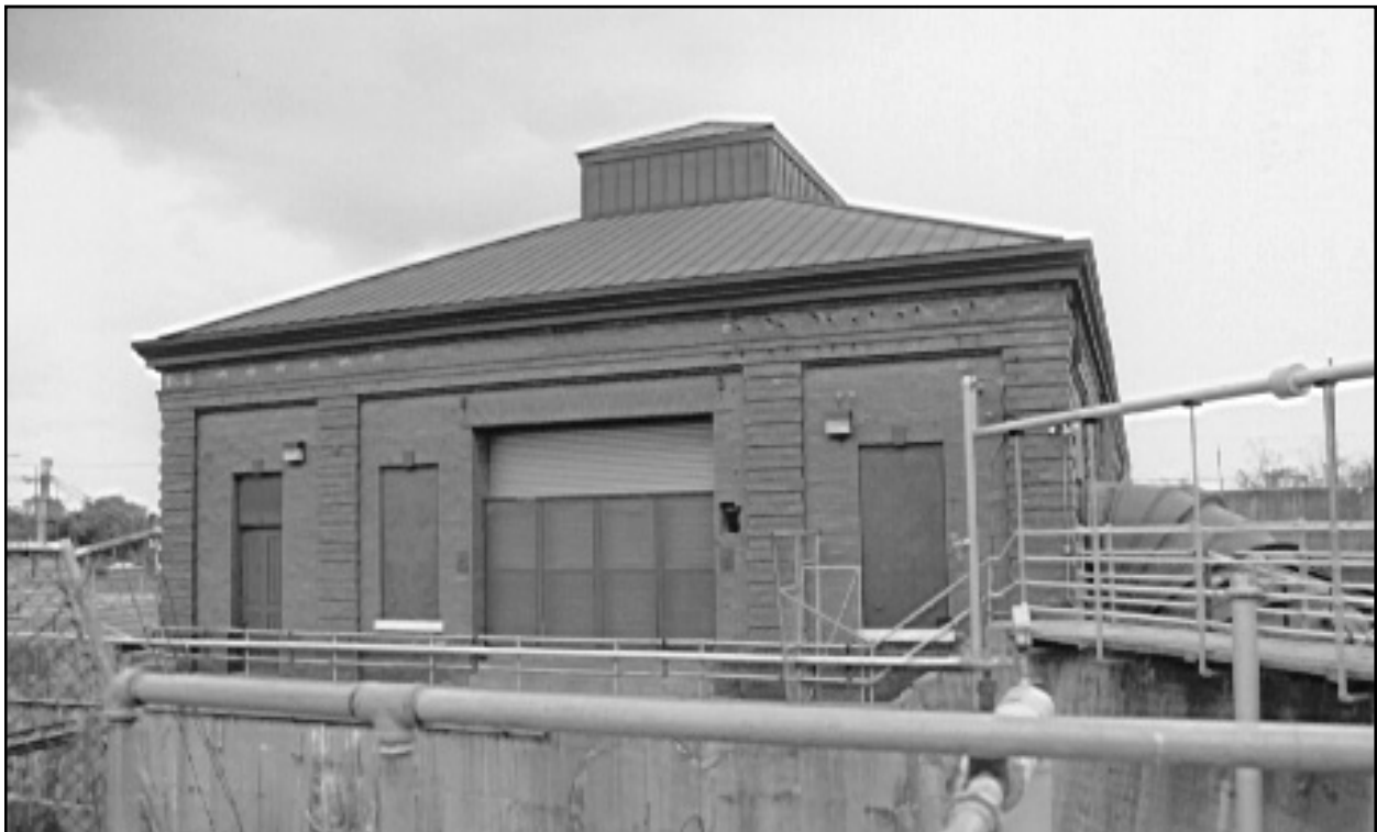
Figure 40. Drainage Pumping Station No. 3, viewed from the northeast.
