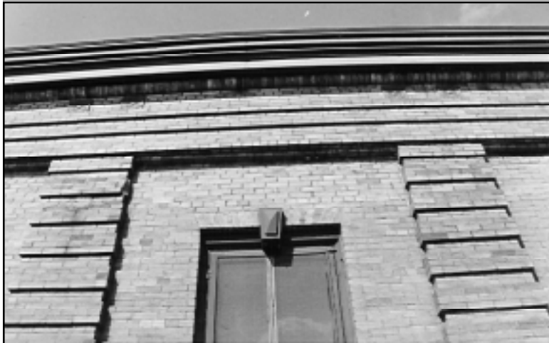
Figure 85. Drainage Pumping Station No. 1. View of upper portion of east facade of building, showing pilasters, wall, and entablature, quarter-round bricks at transition to cornice, and decorative cast-metal false key-stone on window.
