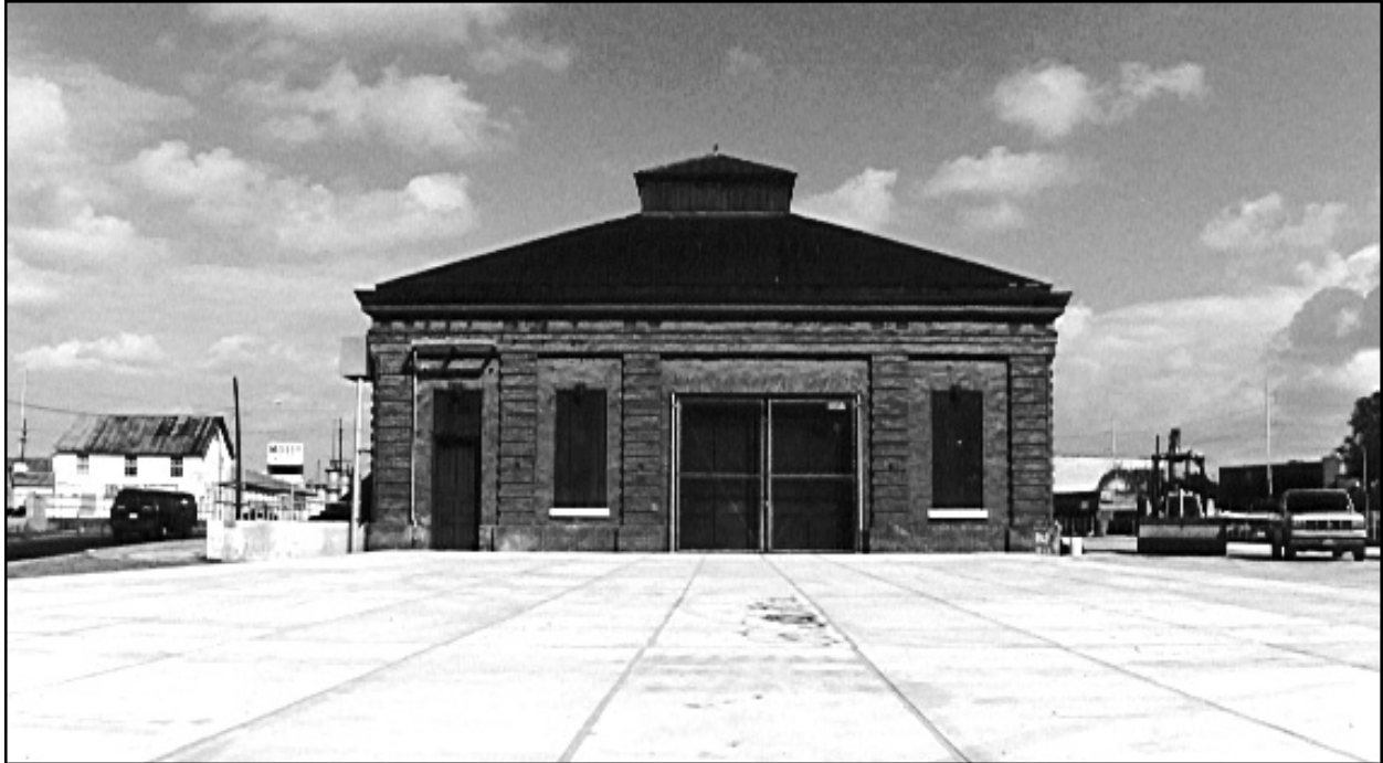
Figure 34. Drainage Pumping Station No. 1. View of south facade, looking north.
