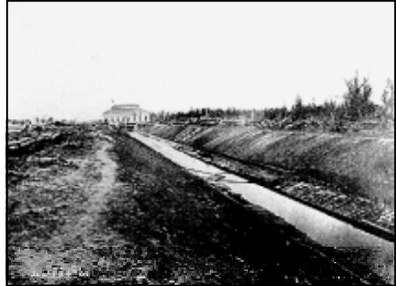
Figure 70. Melpomene Outfall Canal, 1906. The canal was timber lined and the banks graded, 1905-1906. Drainage Pumping Station No. 1 is in the background (From Sewerage & Water Board 1906a).
