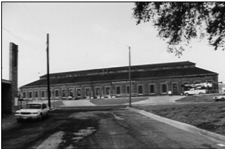
Figure 29. Drainage Pumping Station No. 1. View of east facade, looking west from Martin Luther King Boulevard.
