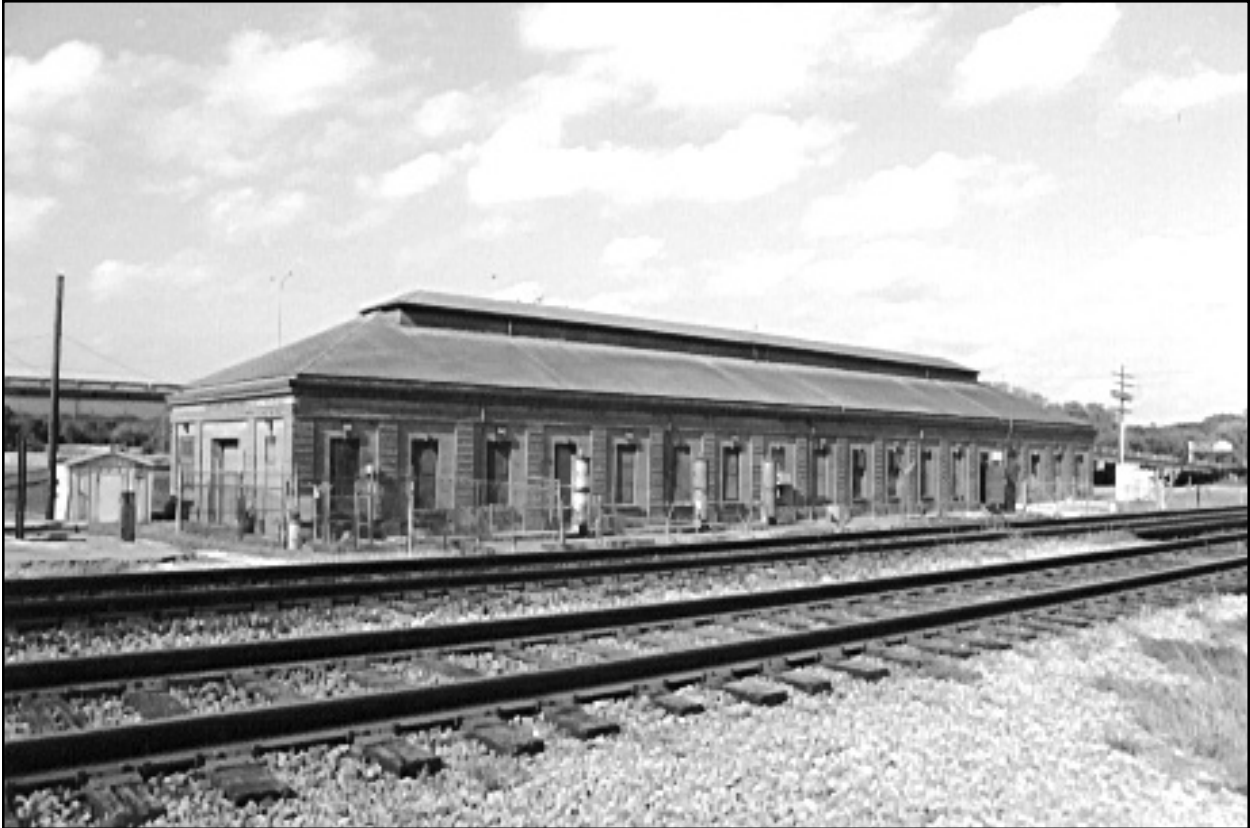
Figure 61. Drainage Pumping Station No. 7. View from the southwest.
