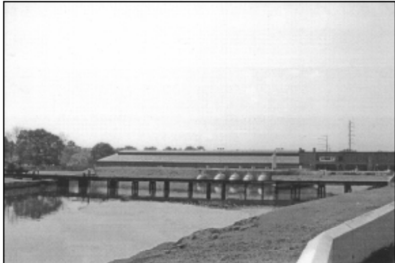
Figure 106. Drainage Pumping Station No. 6 Currently existing station viewed from the north.
