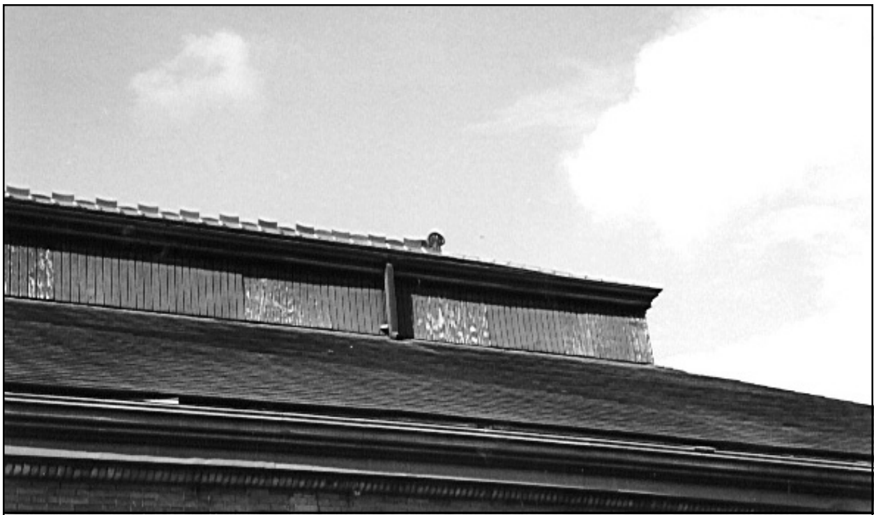
Figure 92. Drainage Pumping Station No. 1. View of the monitor roof peak at the northern end of the building, with terra-cotta crest and finial.
