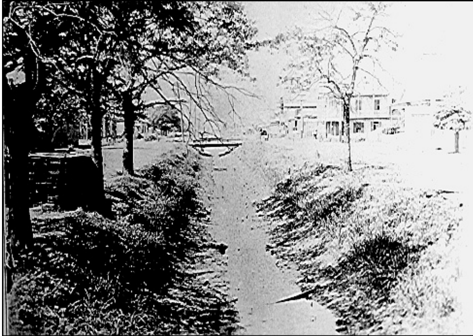
Figure 9. Broad Street Canal after cleaning, 1904 (from Sewerage & Water Board 1904).
