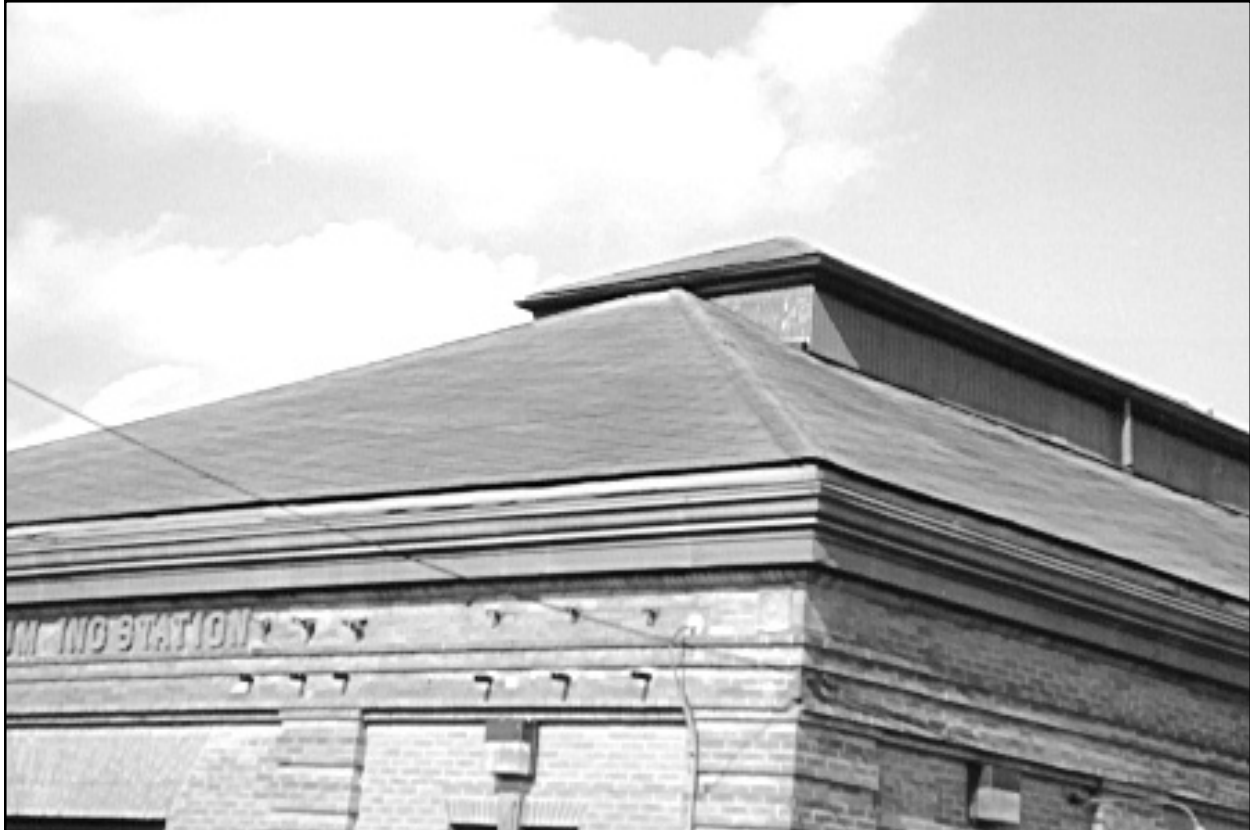
Figure 65. Drainage Pumping Station No. 7. View showing end of monitor.
