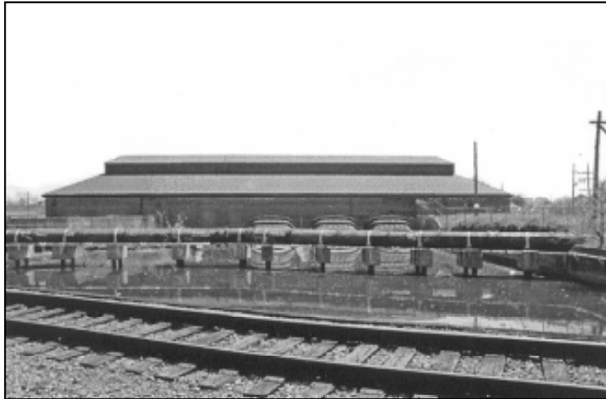
Figure 104. Drainage Pumping Station No. 3. Currently existing station viewed from the north.
